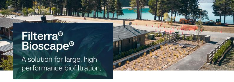
Stormwater360 Filterra® Bioscape® is an engineered, centralised biofiltration system, designed to treat catchments over 10,000m². It uses the patented Stormwater360 Filterra® technology to deliver best-inclass treatment on a small footprint.
