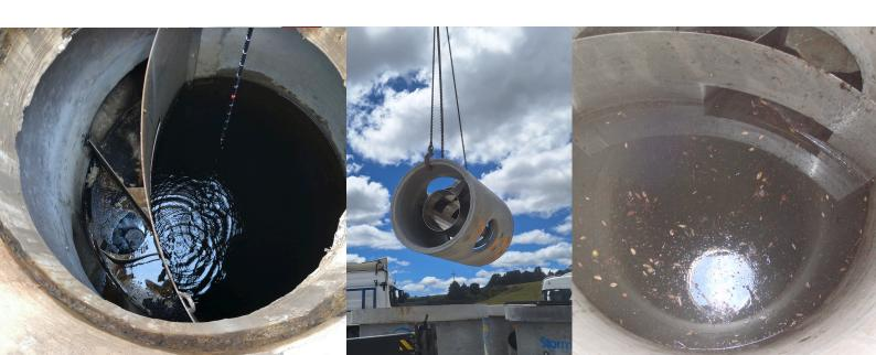
The Cascade Separator™ is the newest innovation in stormwater treatment. This innovative hydrodynamic separator excels at sediment capture and retention while also removing hydrocarbons, litter, and debris from stormwater runoff.
